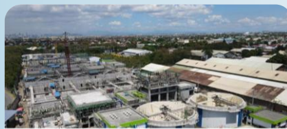
LAS PINAS WRF 61.77% Completed
