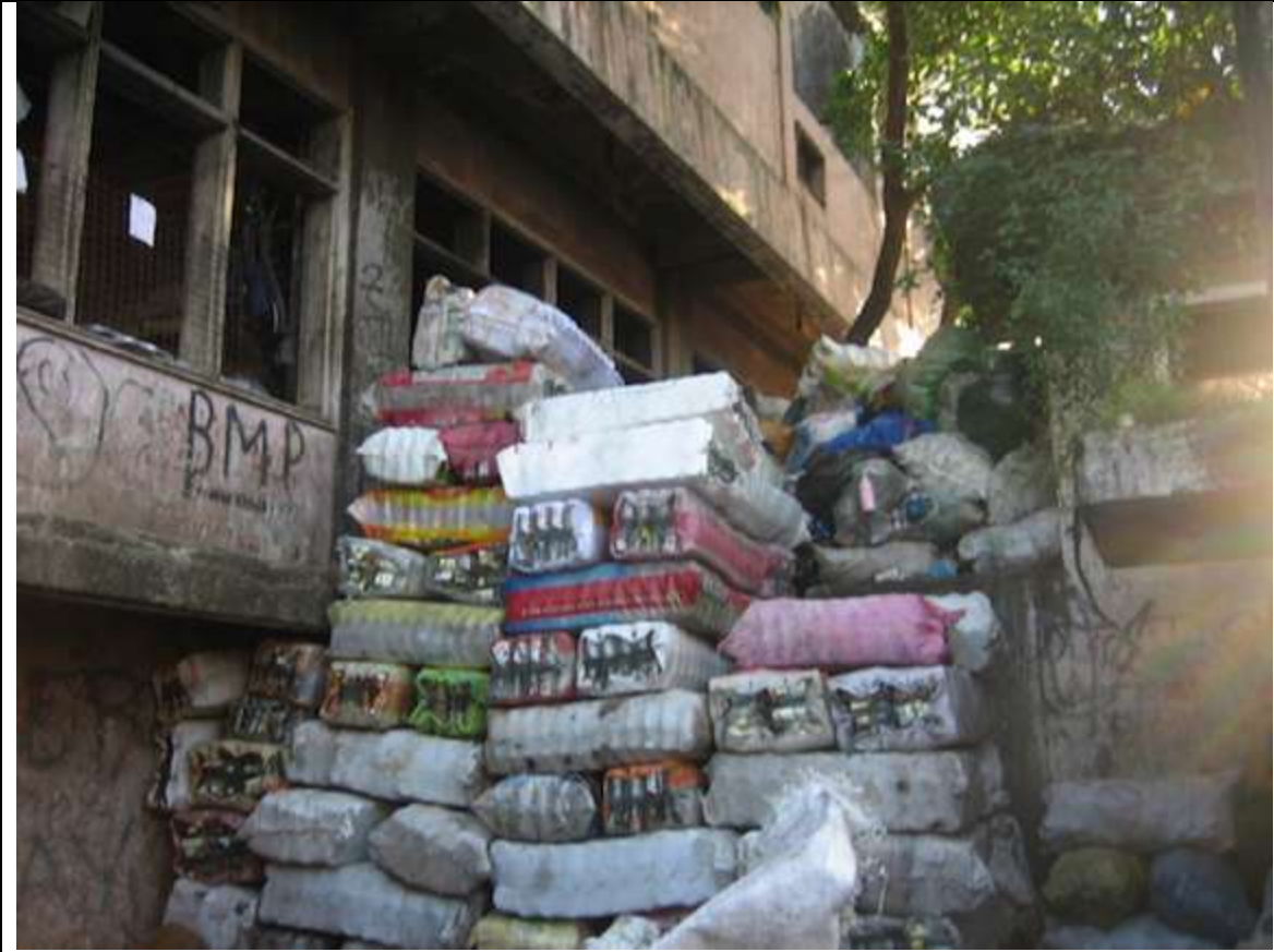
Photo 2. Remaining junk materials to be hauled out.
