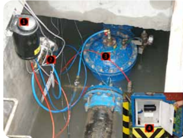
The i2O System is made up of (1) Electronic Controller (2) Pilot (3) Pressure Reducing Valve (4) Sensor.
