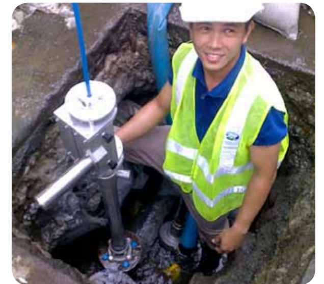
An engineer conducts inspection using the JD7.
