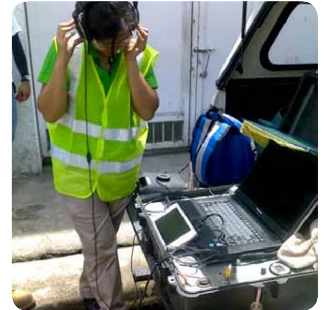
Monitoring pipe condition using JD7 is more efficient.
