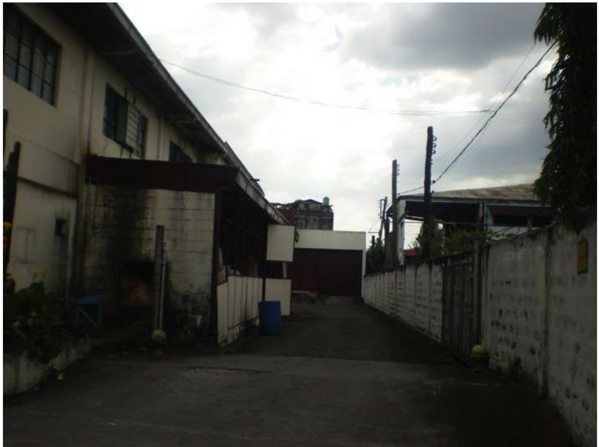
Photo 4. View of the vinyl factory at the central section of the property that is schedule to vacate the property in December 2011.
