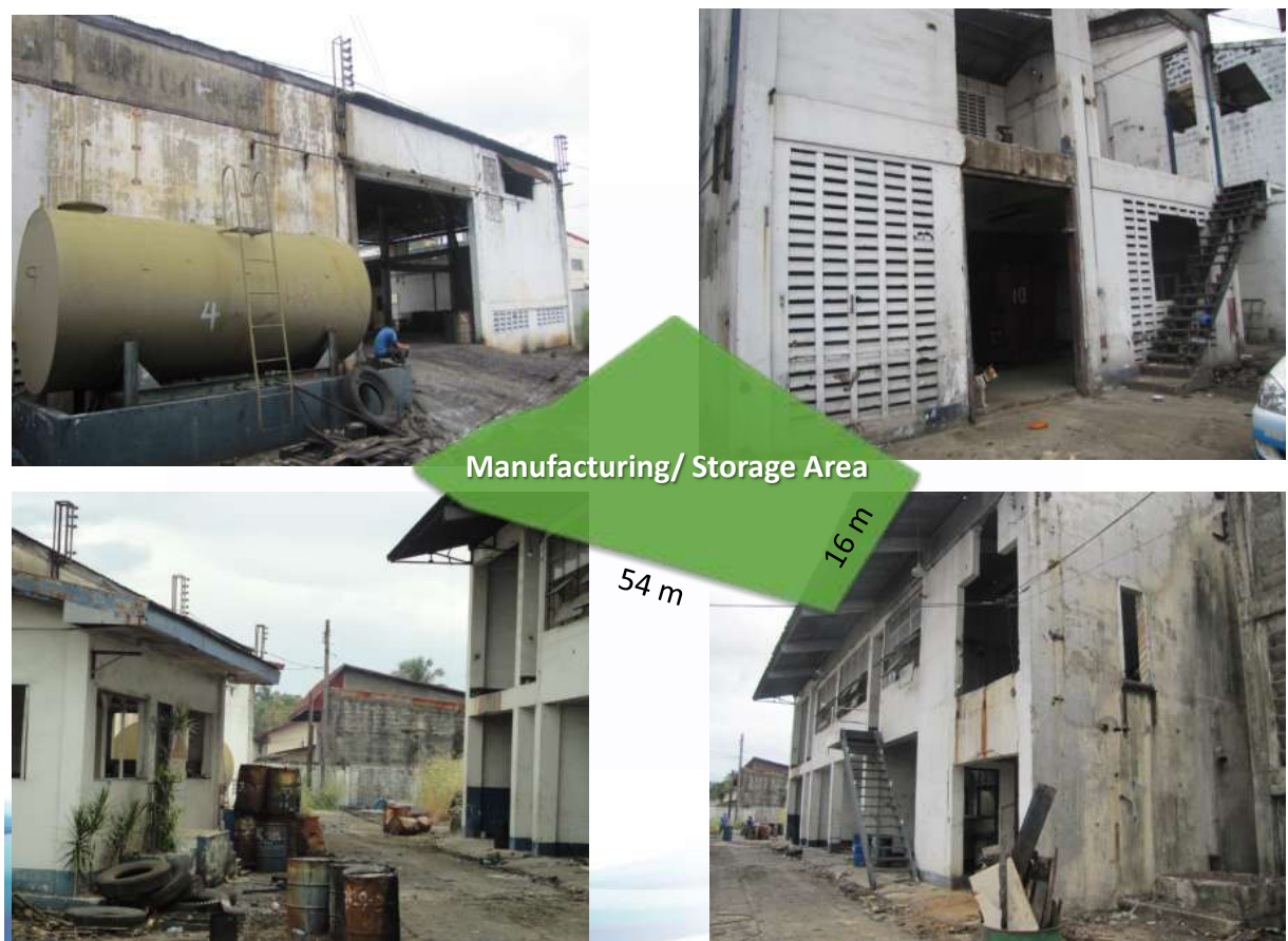
Photo 2. Remaining structures of Kemwerke, former occupant of the site.
